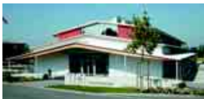
Our international facility in Schenkon, Switzerland
